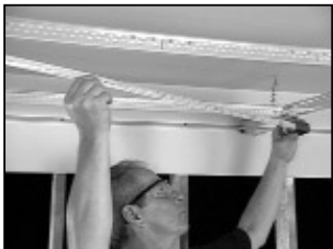
Square the grid by measuring across the diagonal of the grid opening
