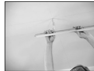
Install first main beam
