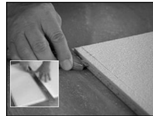
Regular-edge border panels may require field cutting. Cut border panels face up
