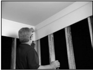
Mark desired height for new ceiling
